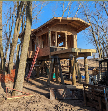
Treehouse being constructed
